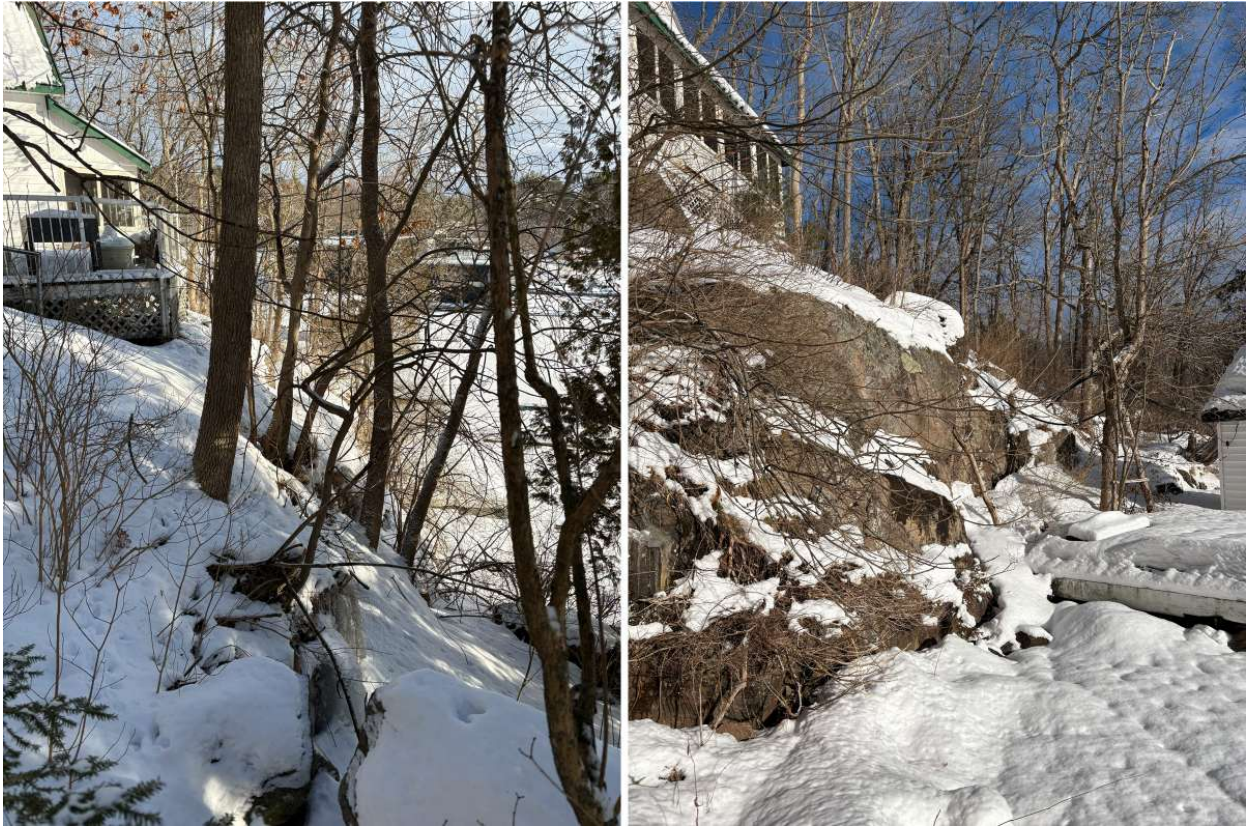
Figure 2. Photos show an example of the terrain of the Shore Road Allowance (aka "Water Street") at 5 Rice Street. The SRA is narrow and treacherous in spots, making it unrealistic and a legal liability as a public thoroughfare.
